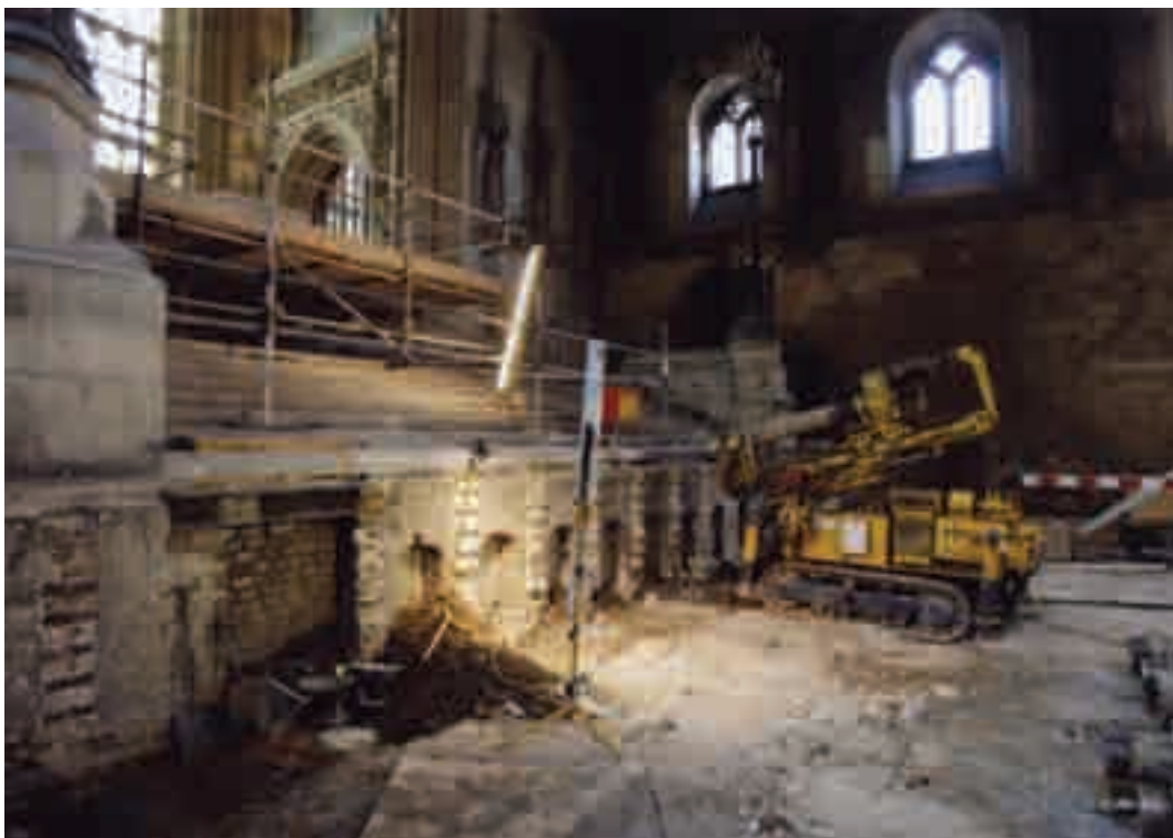
Major conservation work took place in Westminster Hall during the year.
