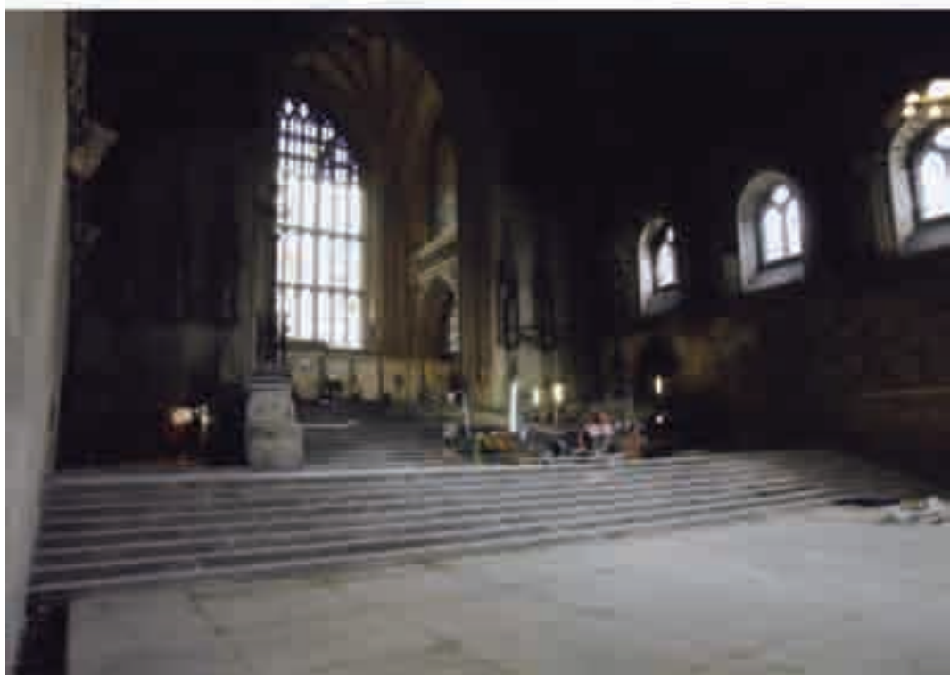
Each flagstone was relaid in its original location.
